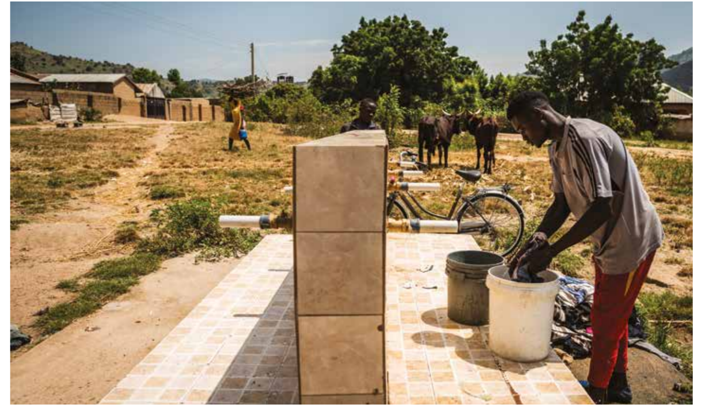
The Tudun Wada Bazza, Michika, community well in Adamawa State was built in 2019 and provides around 3000 people with clean water for domestic use and irrigation. The two collection points, with 12 taps each, have become the center of village life. The photos show views of everyday life: a boy washing his motorbike, another doing the laundry and children filling their cans.
